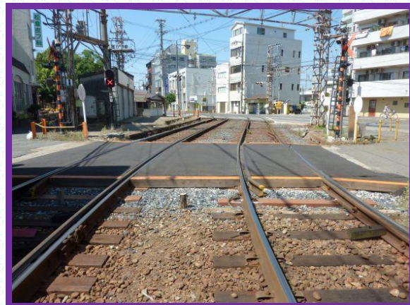
(神ノ木6号踏切道)
